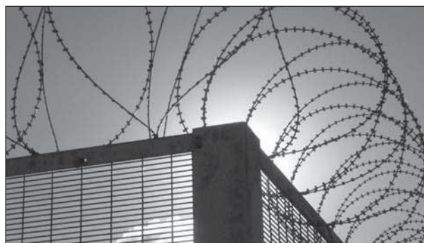
TOP RAIL WITH CONCERTINA RAZOR TAPE ATTACHMENT
